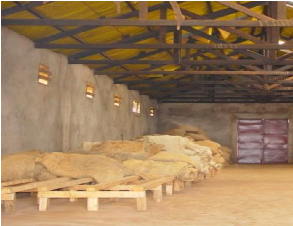
Store equipped with wooden pallets, 15cm above the floor
